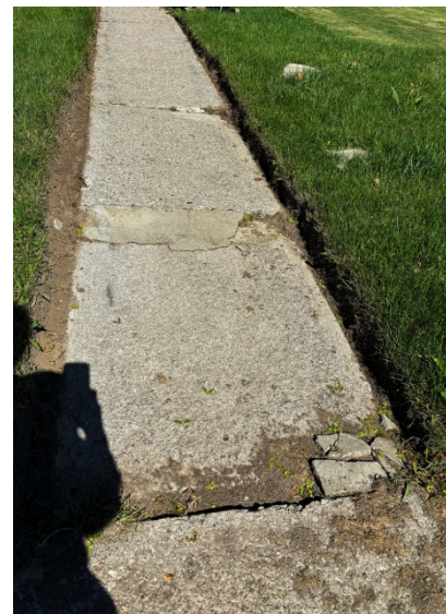
Current condition of walkway from street
